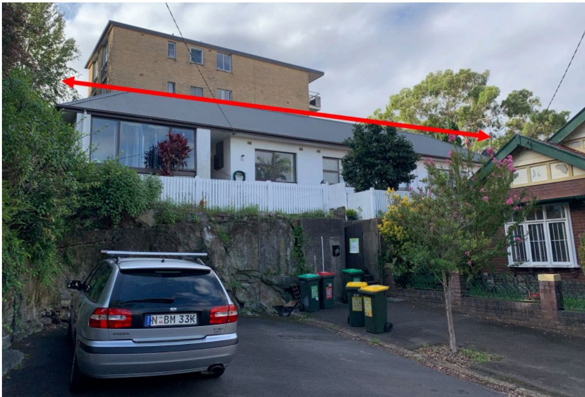
existing Avona Avenue elevation of the site
