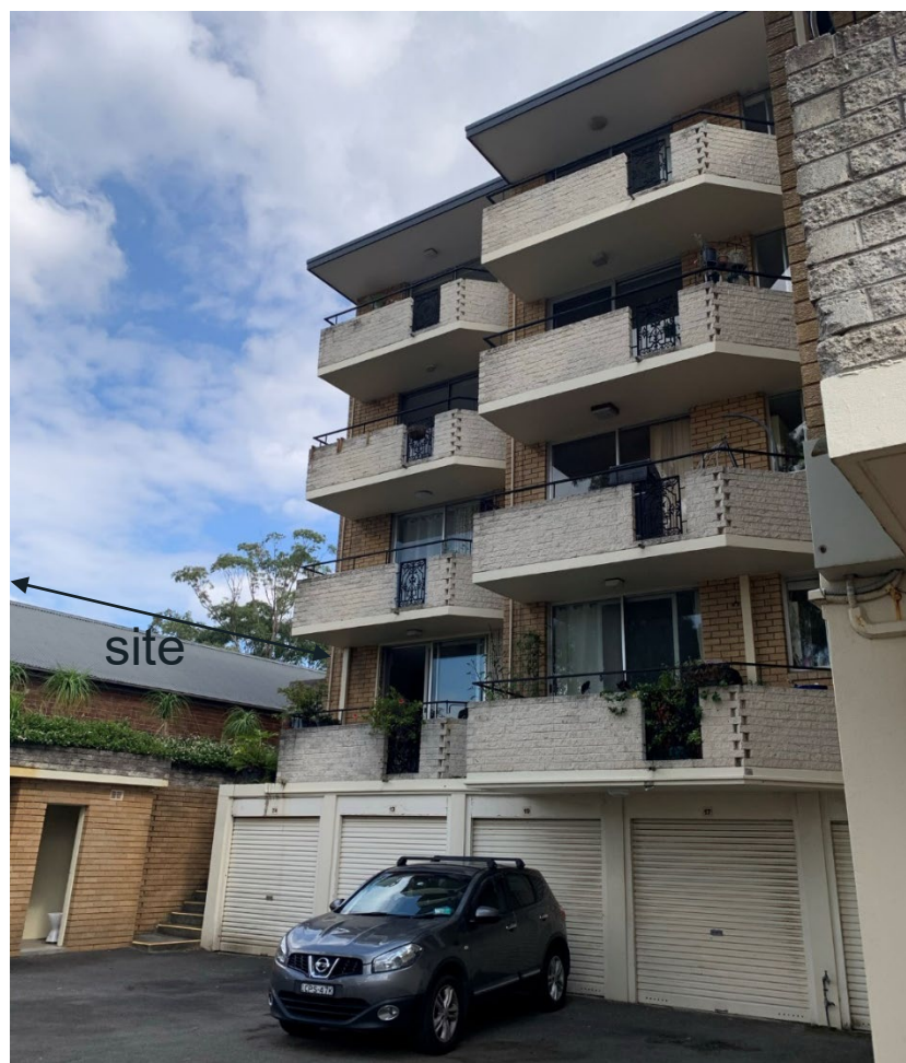
9A Cook Street (east elevation) – subject site is to the south
